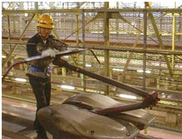
Inspection of pantographs
