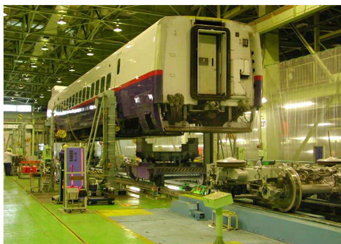
Removing bogies from cars
